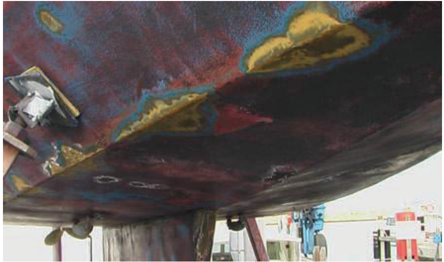
Paint blistered off along weld lines and other random spots.
